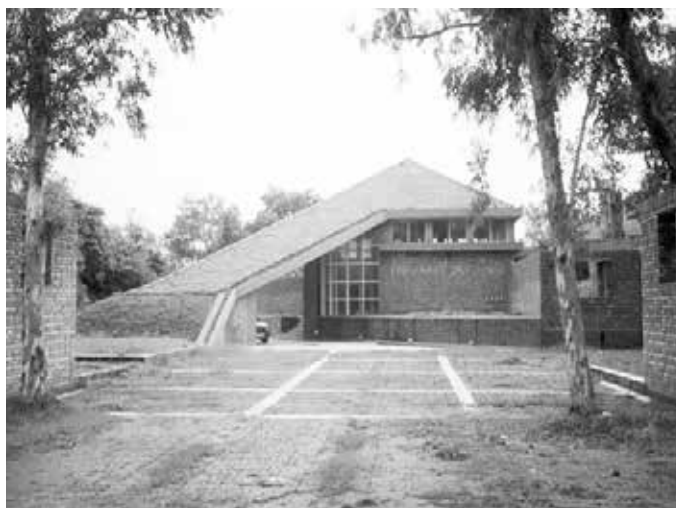
A view of the International Hostel for scholars-in-residence in Gandhi Darshan complex, Rajghat.
